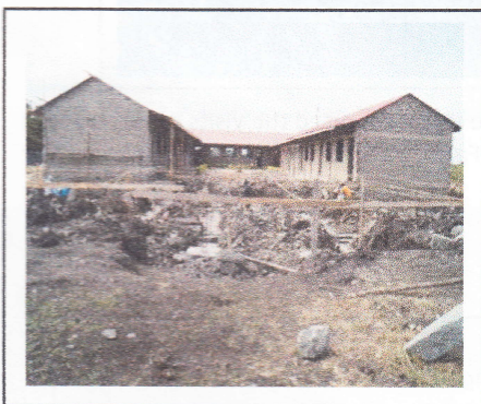
Athi, St. Michaels Primary School, 12 classrooms and foundation setting for the administration block
