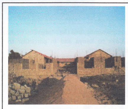
Athi, St Michaels school administration block under construction.
